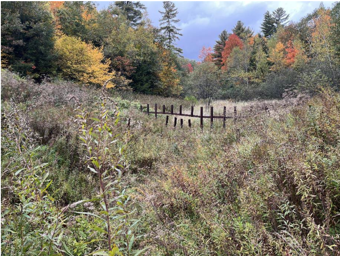
Train rail beaver barrier fence at culvert inlet, (Hydraulics/Scoping site visit photo 10/10/2022)
