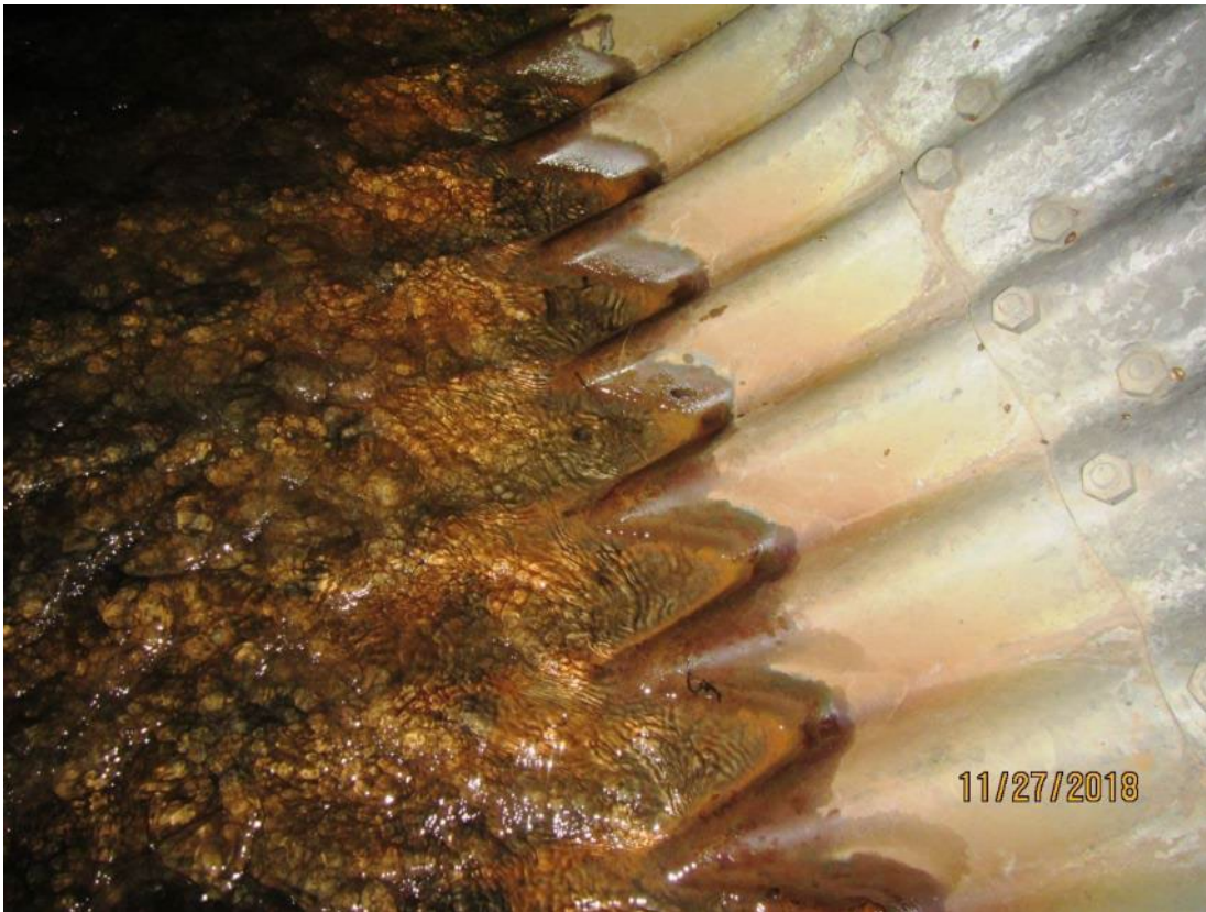
Invert damage, (Inspection finding photo 2018)
